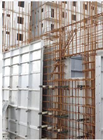
Shear Wall based construction
